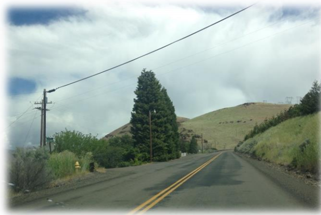
Exhibit 6-3. Example of Scott Canyon Road
