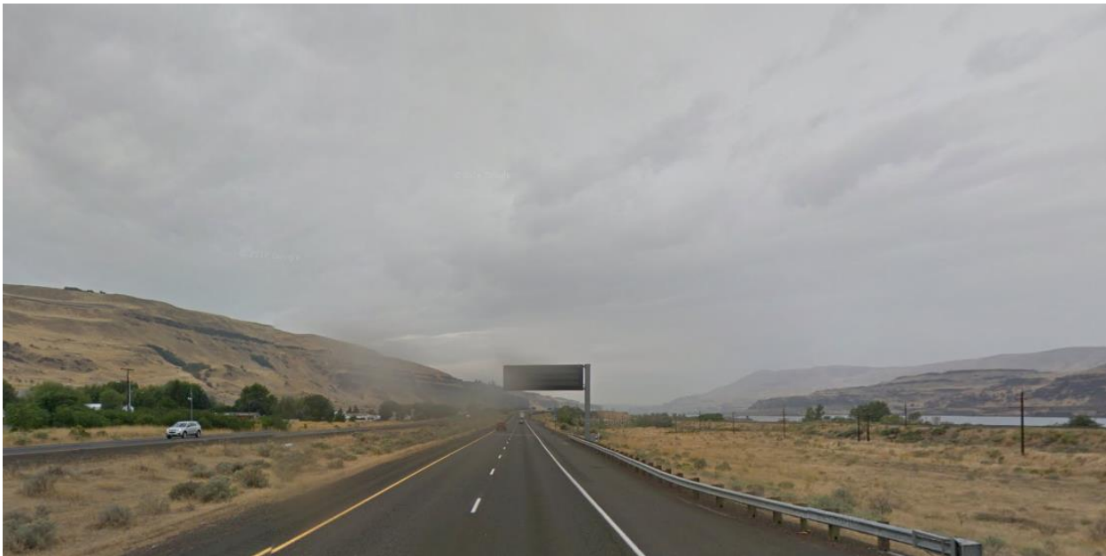
Existing I-84 westbound variable message sign at Rufus
