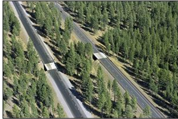
Figure 2. The project developed wildlife-only passage structures for both the northbound and southbound corridors. Source: ODOT
