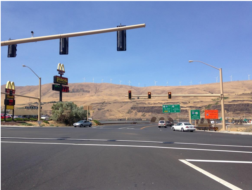
New traffic signals at Biggs Junction, July 2015
