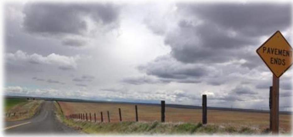
Exhibit 6-4. Blagg Lane, East of Raceway
