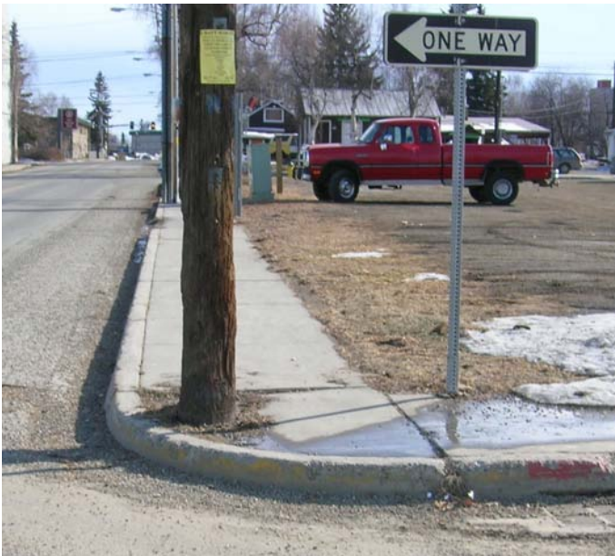
Lack of curb ramps and obstacles in the sidewalk limit accessibility for all users
