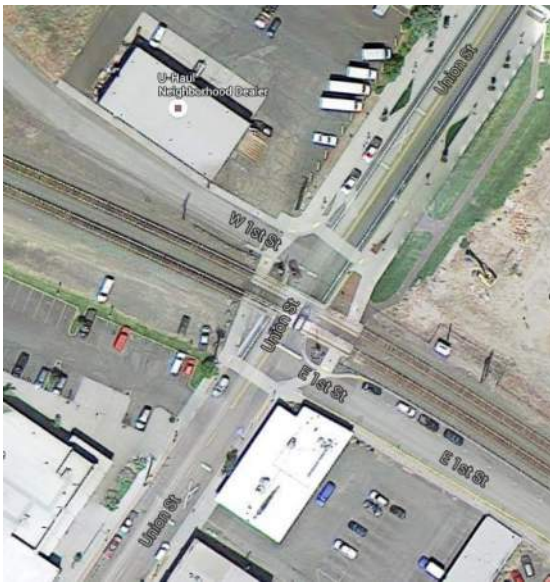
Exhibit 4-1. UPRR Railroad Crossing at Union Street
