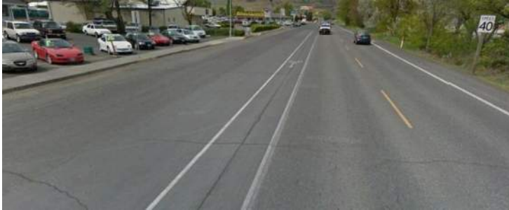
Exhibit 5-2. 6 th Street 700 feet north of 6 th Street/Snipes Street intersection
