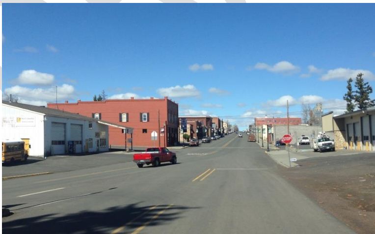
Exhibit 6-3. Sidewalk gap on OR 206 at Main Street in Condon
