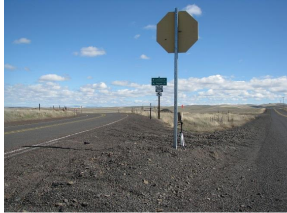
Exhibit 6-2. Restricted Sight Distance at OR 206/Lonerock Road
