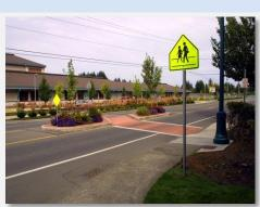
A raised median island provides a protected area in the middle of a crosswalk for pedestrians to stop while crossing the street. These refuges allow pedestrians to cross one direction of traffic at a time. Pedestrian refuges are often used in areas with high traffic volumes and/or at locations with a crash history involving pedestrians.
