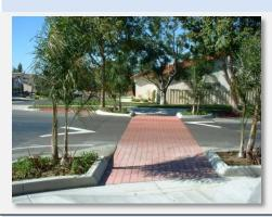
A raised crosswalk is raised higher than the surface of the street to give motorists and pedestrians a better view of the crossing area. A raised crosswalk is similar to a speed table and are often marked and signed for pedestrian crossing. Raised crosswalks are often used in areas with low speeds where people and difficulty crossing the street.
