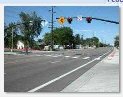
A HAWK is a pedestrian-activated signal that is unlit when not in use. When activated the signal begins with a yellow light alerting drivers to slow and then a solid red light appears requiring drivers to stop while pedestrians have the right-of-way to cross the street. HAWKs are often used on wide roadways where midblock crossings are difficult.
