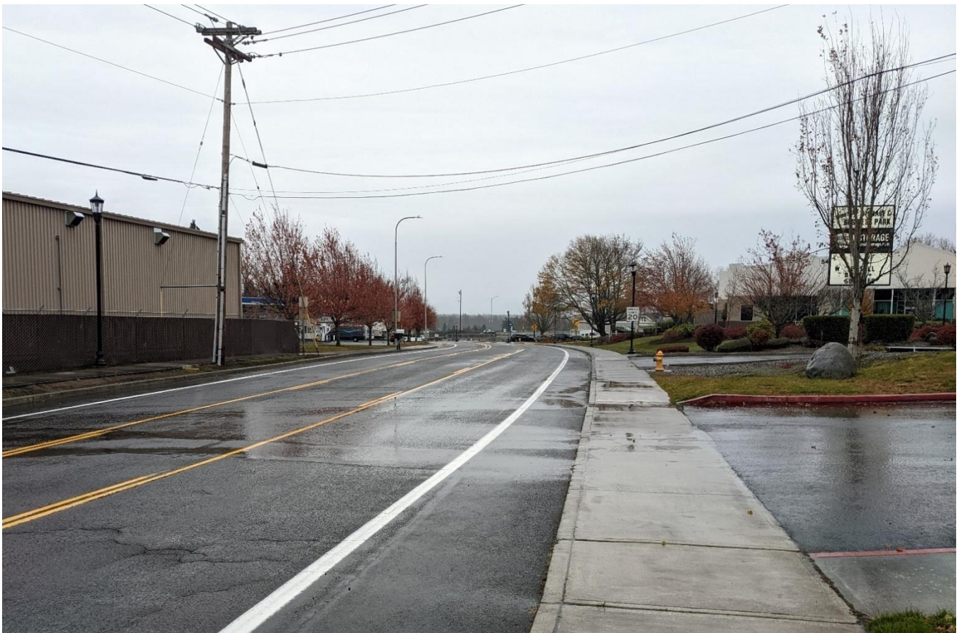
Figure 8: Typical existing conditions in the Commercial context zone
