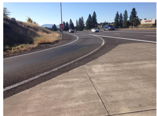
Crater Lake Parkway Crossing Between Campus Trail and Biehn Street
