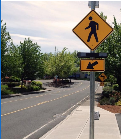
Rectangular Rapid Flashing Beacon (RRFB) at "B" & "C" Avenue
