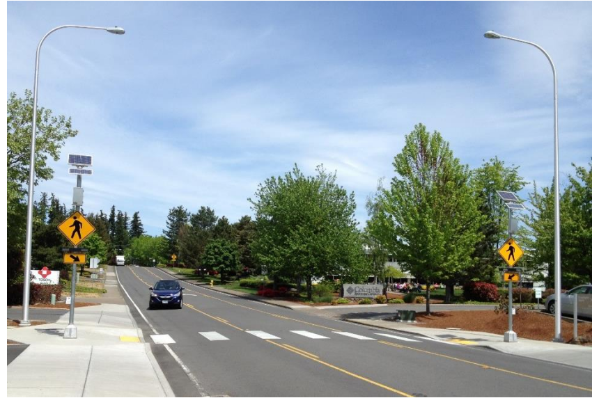
Enhanced Pedestrian Crossings (RRFB)
