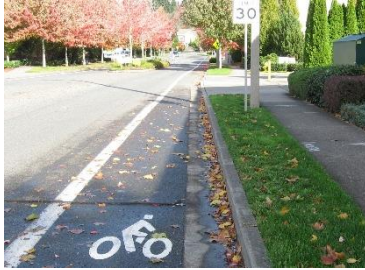
Curbed Roadway with Bike Lane and Sidewalk
