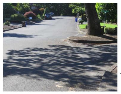
This curbed island on Devonshire at Doncaster extends into the roadway. The City may wish to consider the installation of an OM3-R object marker in this island. An OM3-L object marker for traffic in the opposite direction would be optional.
