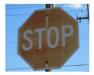
STOP sign at Exeter and Portland that is faded and might have poor retroreflectivity.
