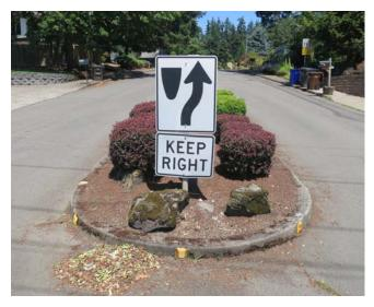
This Keep Right symbol sign on Ridgegate at Oatfield, should have a minimum mounting height of five ft from the pavement to the bottom of the sign. The KEEP RIGHT plaque is not required. An alternative would be a Type 1 object marker (see page 135 in the MUTCD).
