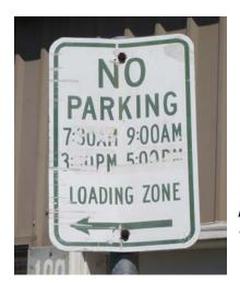
This sign is located on Berkeley just west of Portland. It is in poor condition, and when it is replaced, it should have red legend on a white background.
