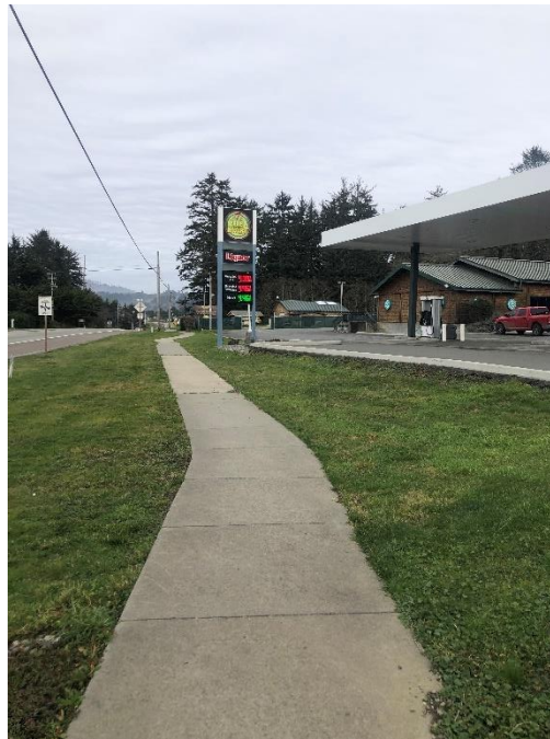
Figure 35. Sidewalk Along Bus Stop
