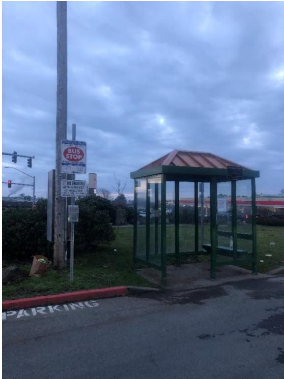
Figure 39. 5 th Street/Bankus Park Bus Stop
