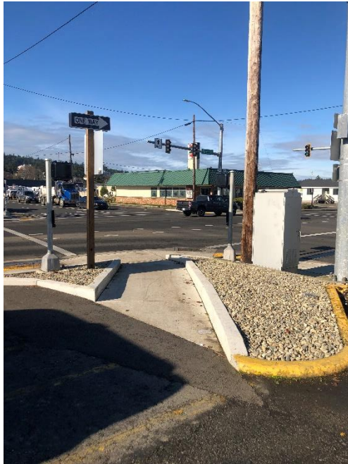
Figure 10. Curb Ramp Access to Sidewalk
