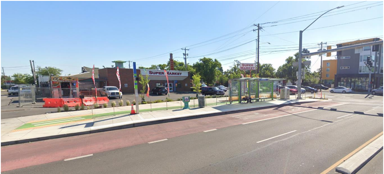
Figure 23: Example Bus Pullout Treatment (Portland, Oregon)
