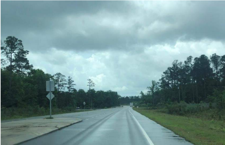
Figure 10. Paved Shoulders on Mount Misery Road and Cedar Hill Road Provide the only On-Street Bicycle Facilities in Navassa
