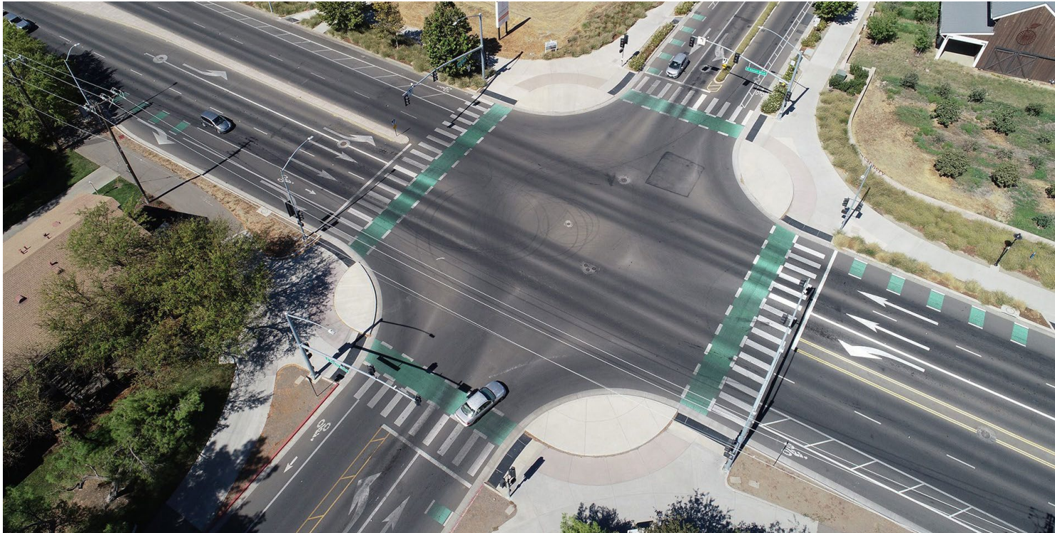
Protected intersection in Davis, CA
