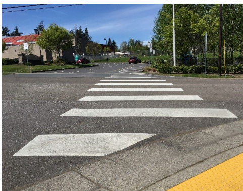
Crosswalk marked with painted striping
