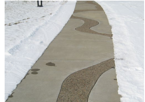
Concrete and aggregate paving
