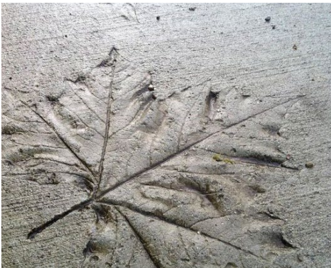
Stamped concrete paving
