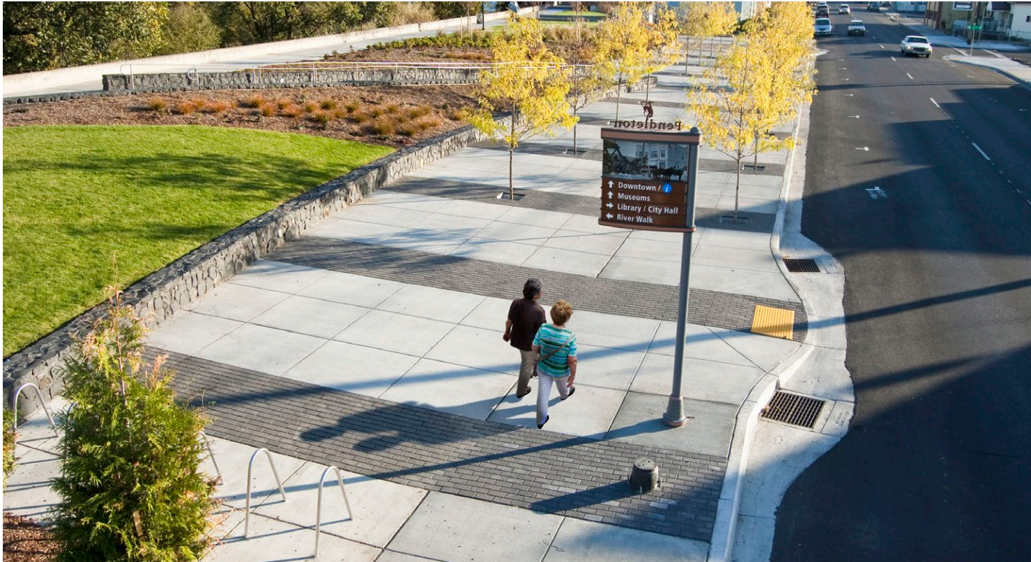
Unit pavers and concrete paving in Pendleton, OR
