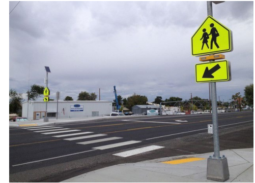
Crossing with rectangular rapid flashing beacon
