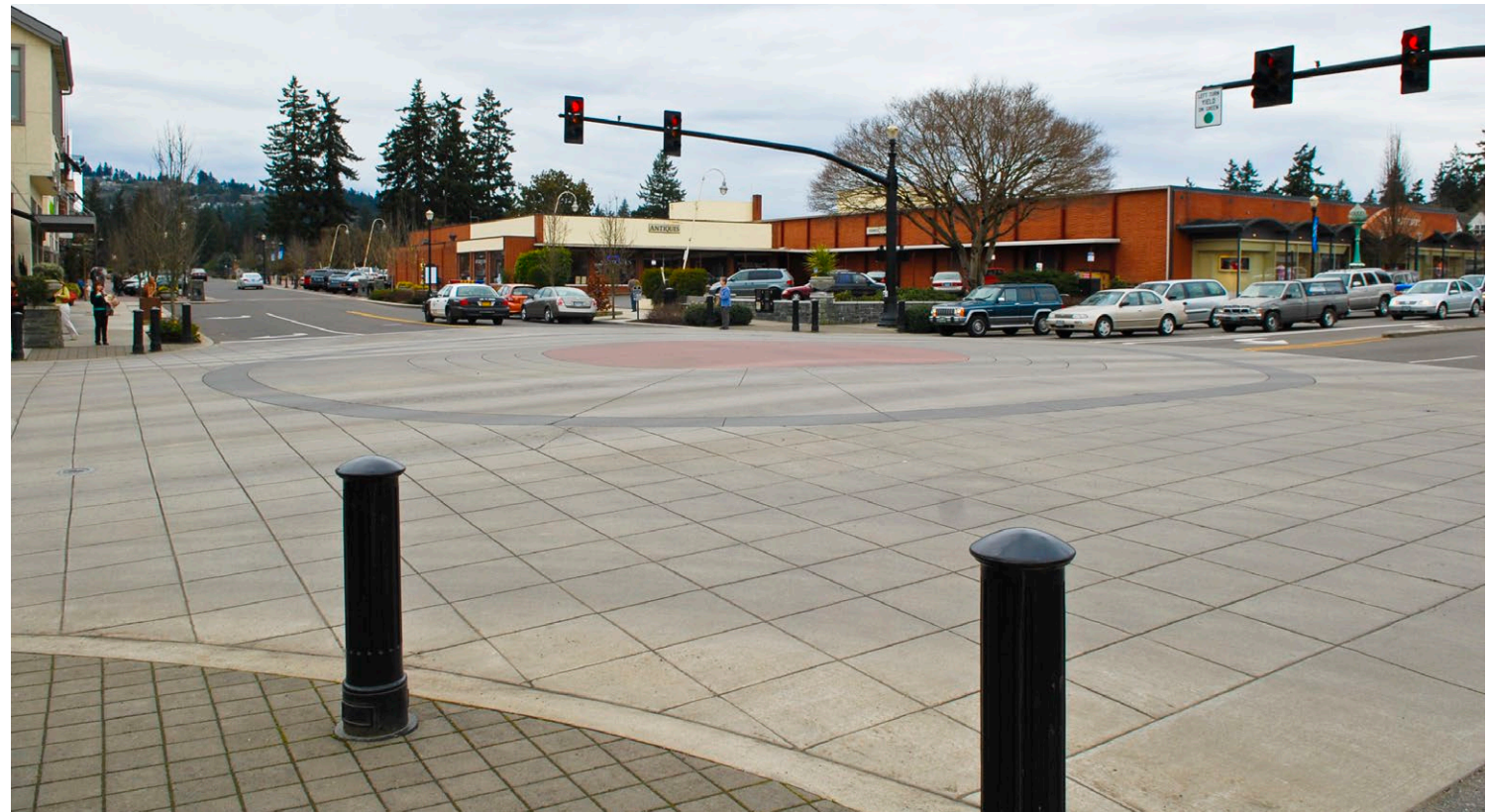
Change of color and materials mark this raised intersection
