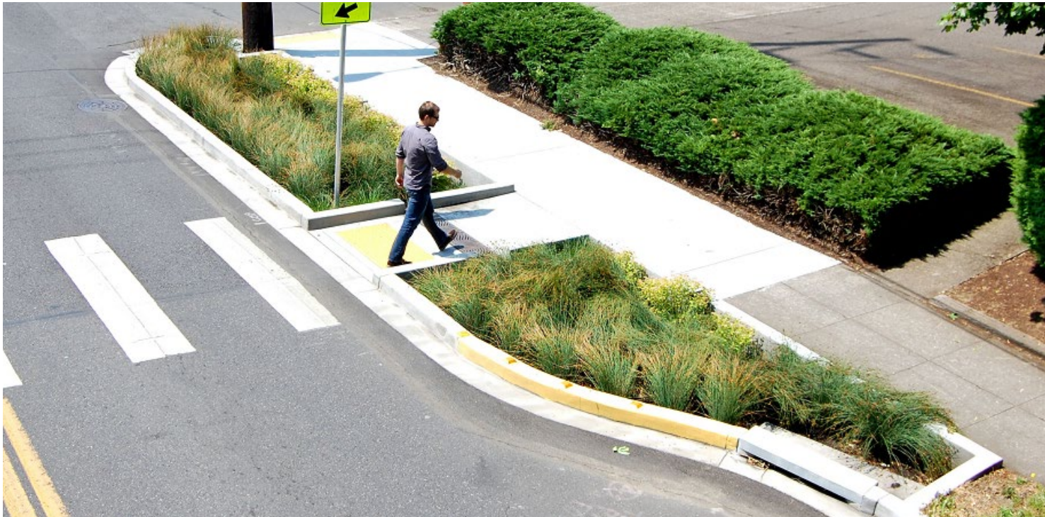
Bulb-out with stormwater facility and crosswalk
