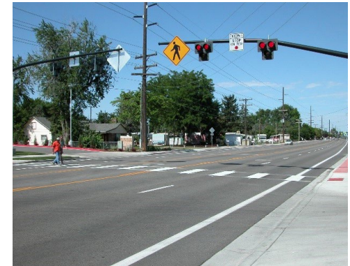
Crossing with pedestrian hybrid beacon
