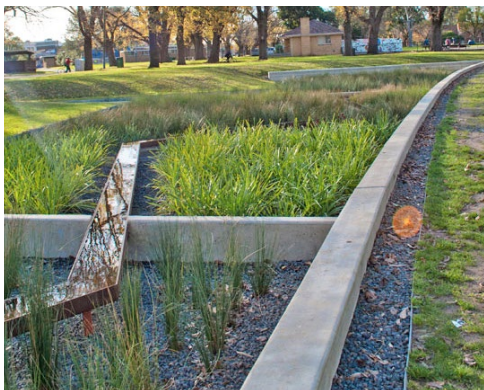
Artistic rainwater conveyance in Melbourne, Australia
