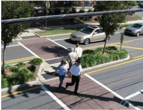
Brick, striping, signage and planters to indicate crossing
