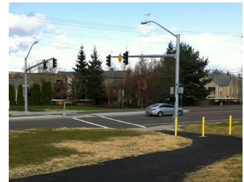
Pedestrian signal at mid-block crossing
