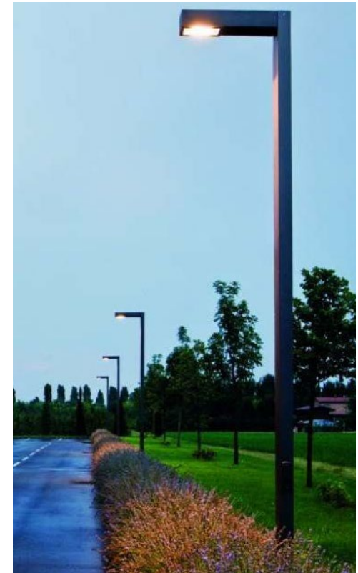
Modern light fixture
