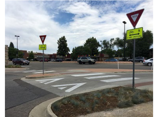
Raised crosswalk leading to pedestrian refuge island
