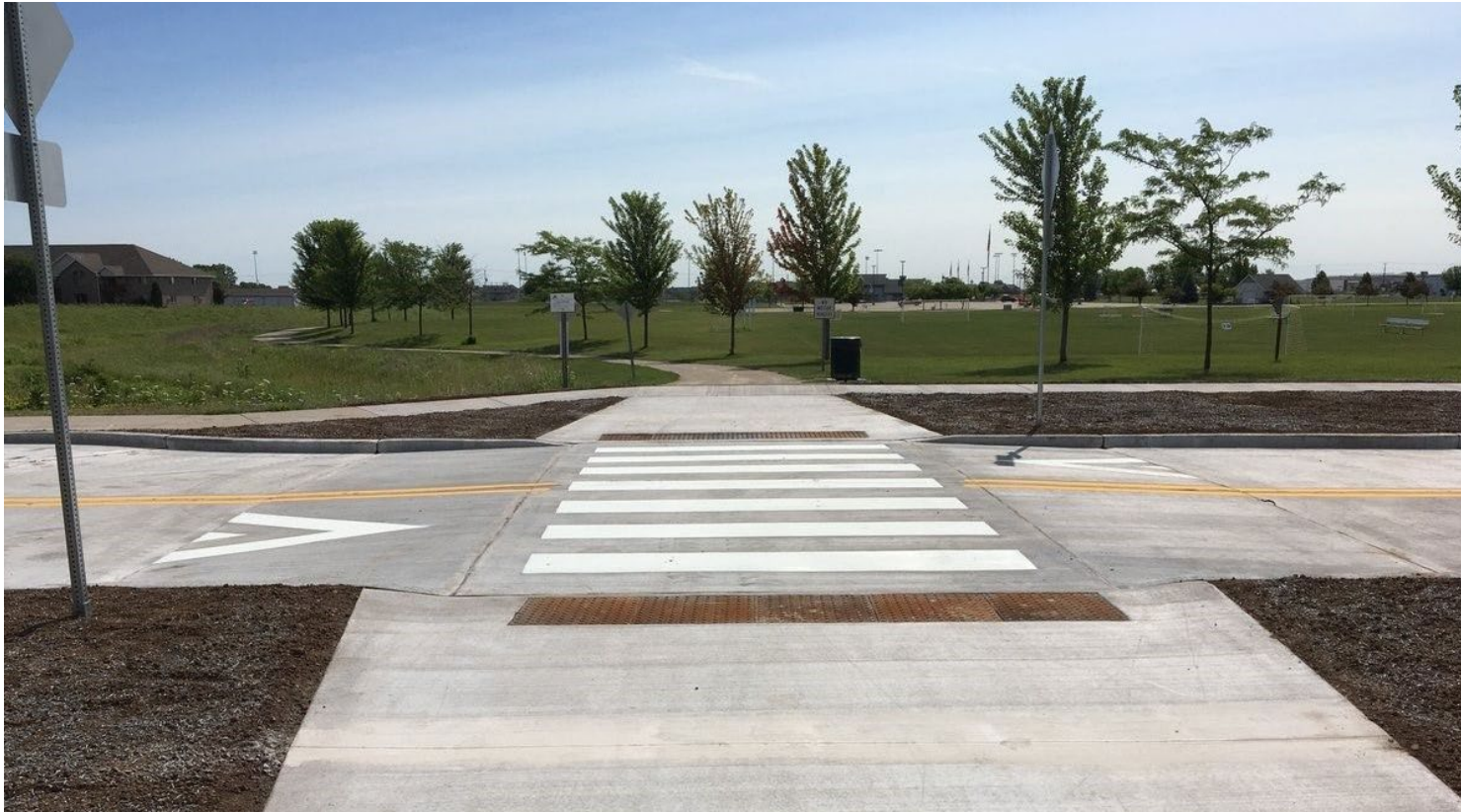
Raised mid-block crossing for a multi-use path in Appleton, WI
