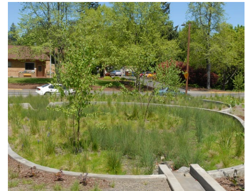
Tiered rainwater basin
