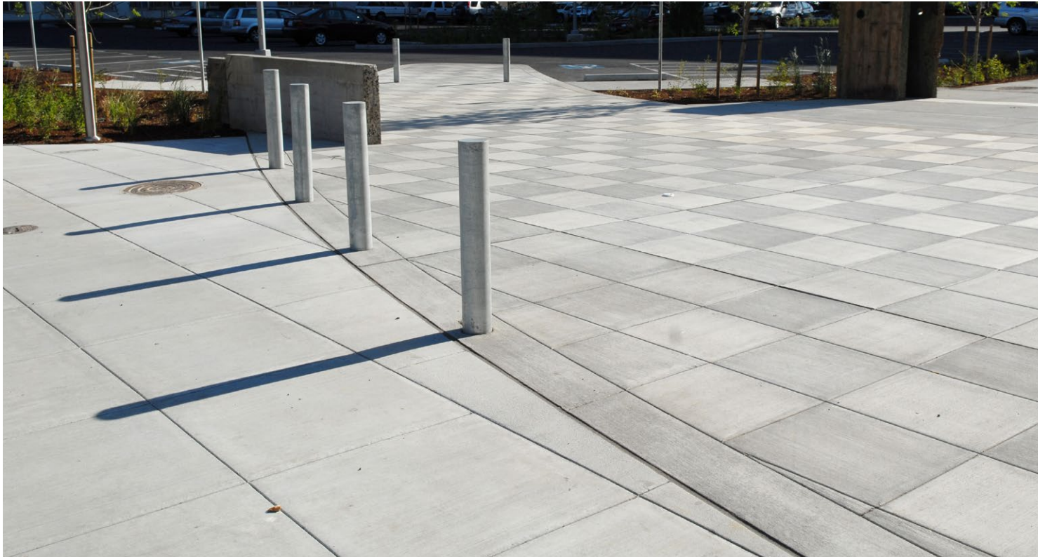
Scored concrete paving
