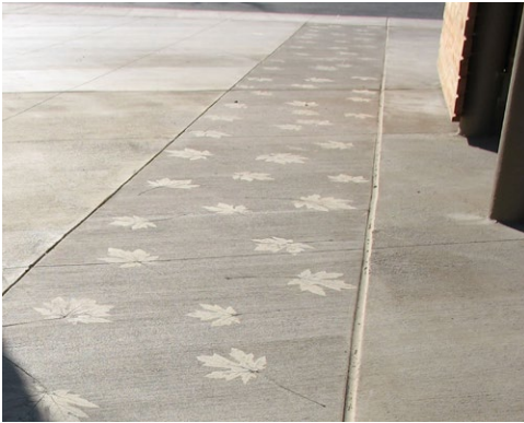
Stamped concrete paving
