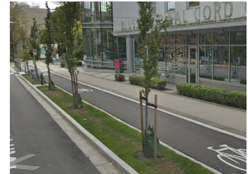
Stormwater tree trench in Vancouver, BC (source: City of Vancouver, BC)
