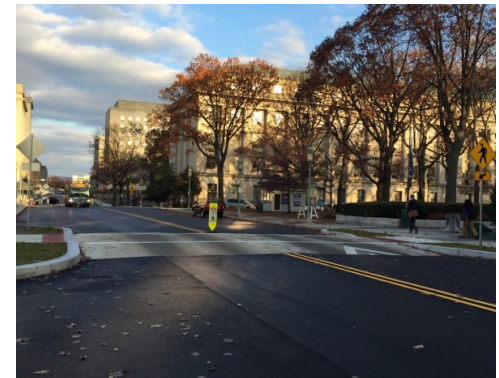
Raised crosswalk with curb extensions (source: PDOT)
