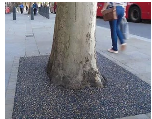
Flexi-Pave porous rubber surfacing (source: KBI UK)
