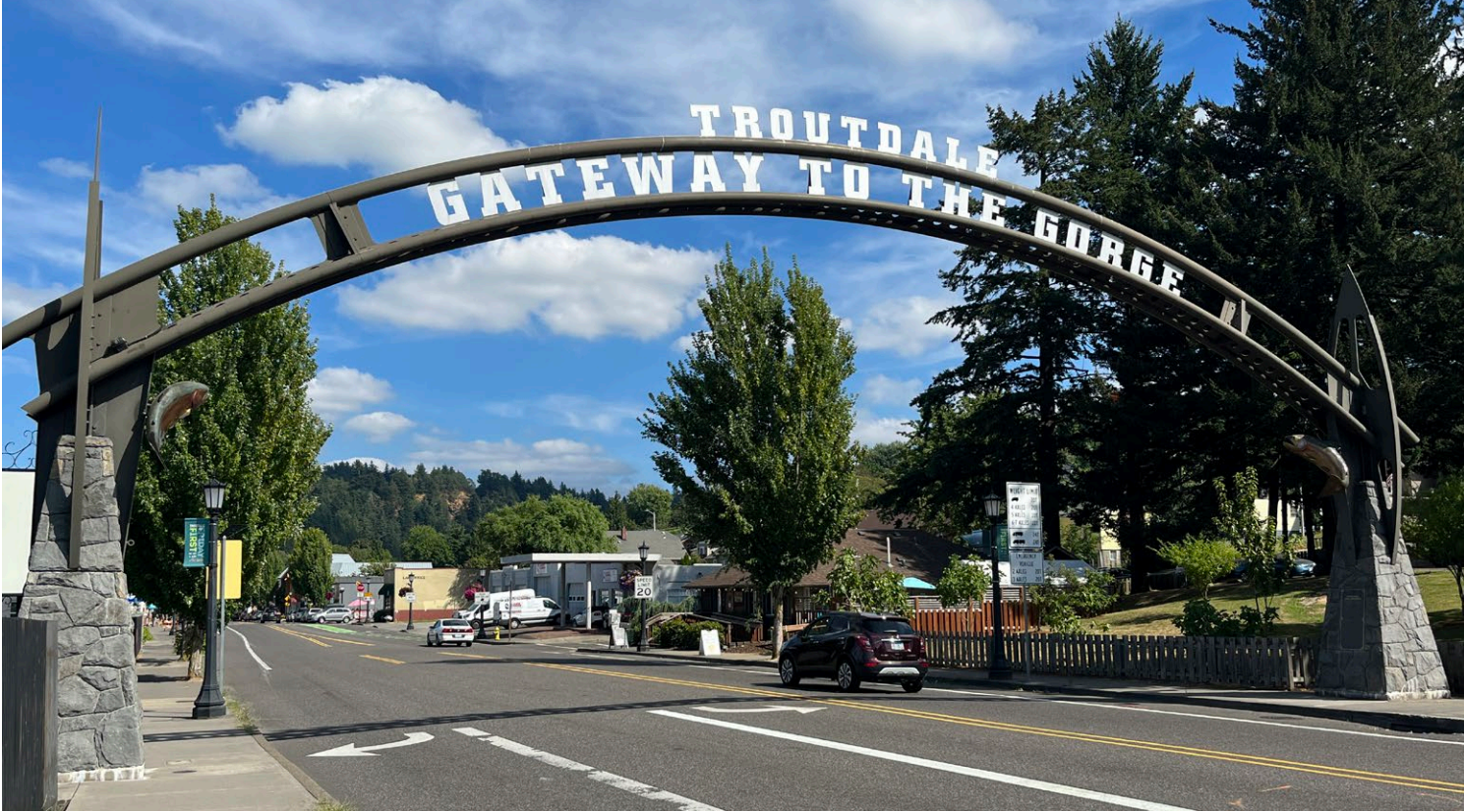
Existing gateway arch in Troutdale
