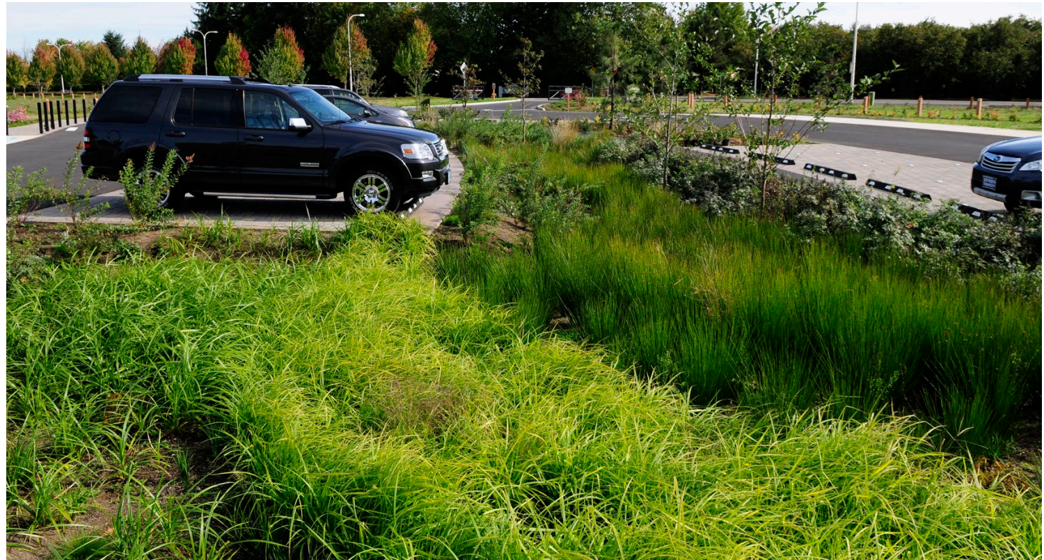
Permeable paving parking stalls at Graham Oaks Nature Park in Wilsonville, OR
