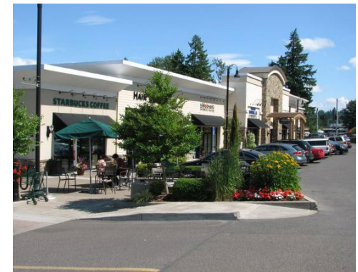
Seating area located in curb extension
